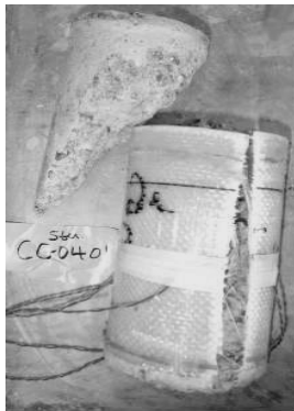
Figure 2: Failure of concrete-filled GFRP tubes
