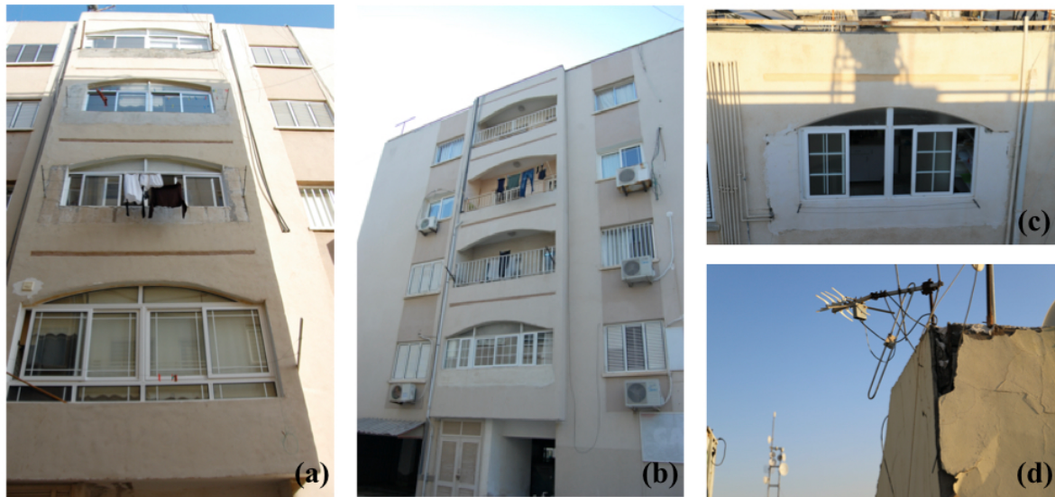
Fig.13. (a) Kitchen balconies and double-glazed, aluminium-framed window systems installed by occupants; (b) wall-mounted A/C systems installed on building envelope; (c) kitchen balcony closure on upper-floor flat; (d) structural failures in junction details between columns and beams on roof.
