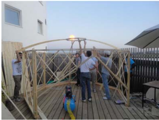
Fig 2: Assembly of the children's shelter.
