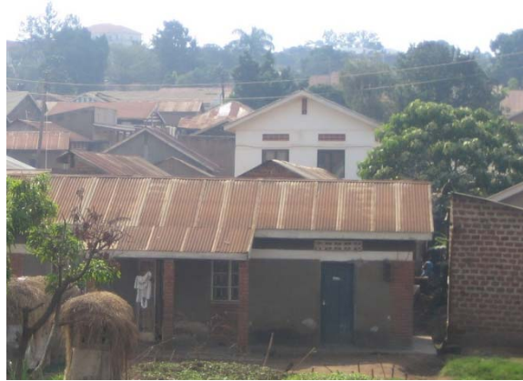
Figure 1. Low-income housing and slums.
