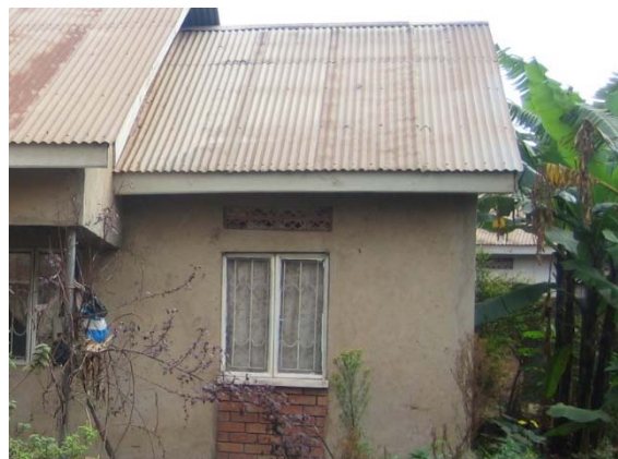
Figure 2. Permanent ventilators on windows and doors
