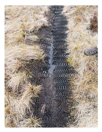
**FIGURE 5** Area of failed track in a rutted section.
