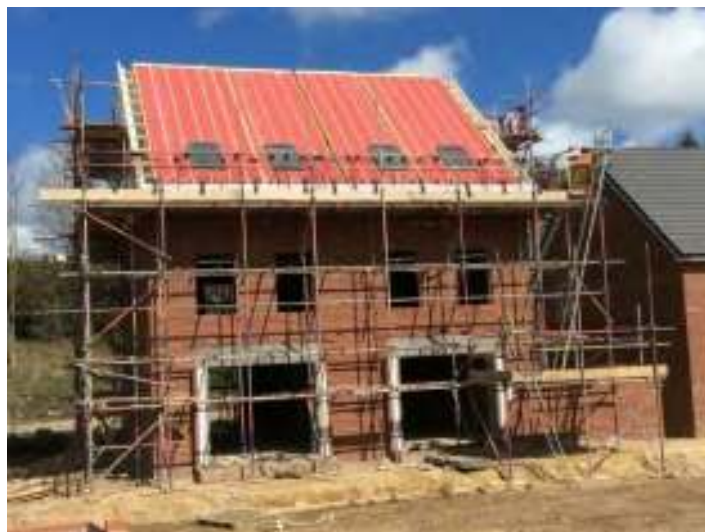
Figure 7: Dwelling awaiting roof tiles.
