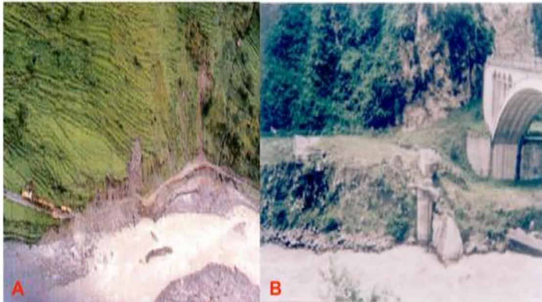
Figure 3.14 The washed away portion of Nepal-China (Kodari) Highway damaged by 1981 GLOF, B. Damaged pier of the old bridge by 1981 GLOF and New bridge at Kodari highway (ICIMOD, 2001)
