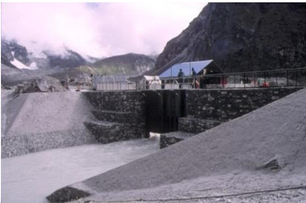
Figure 6.3 Constructed dam and water sluice gate in Tsho Rolpa glacial lake reduction
