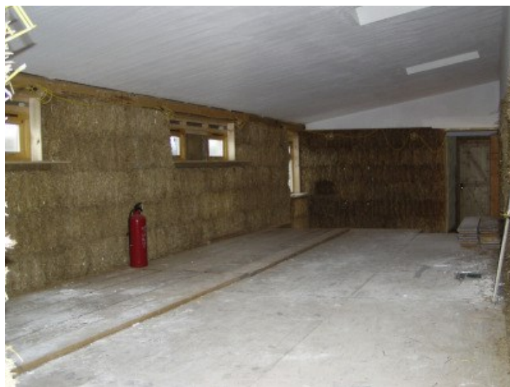
Fig. 7: Load-bearing straw bale wall under construction (Walker et al. 2016).
