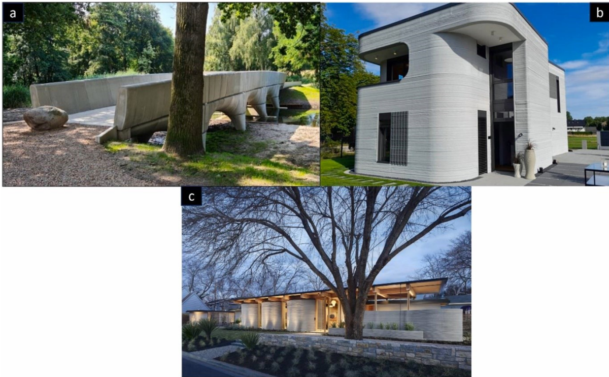
Fig. 12: Examples of projects based on 3DCP: (a) Bridge, Nijmegen, the Netherlands (PERI 3D Construction); (b) Two storey house, Beckum, Germany (PERI 3D Construction); (c) House Zero, East Austin, USA, 2022 (ICON Build).
