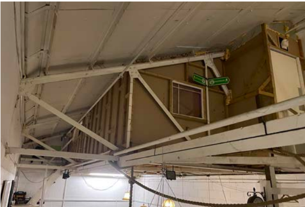
Pitched roof on the metal truss
