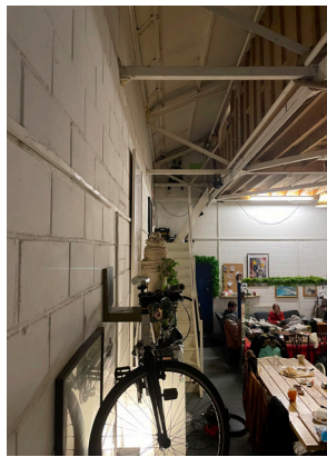
Internal finish of blockwork
