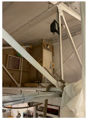
Towards Estelle's room
