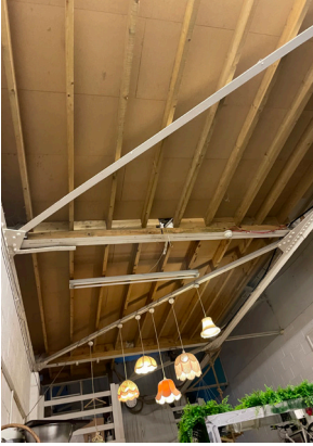
Timber floor joists
