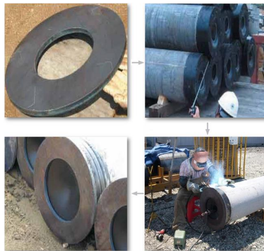
Figure 1. Ext composite pile: (a) extended steel plate; (b) pile dimension check; (c) welding connection; (d) Ext pile
