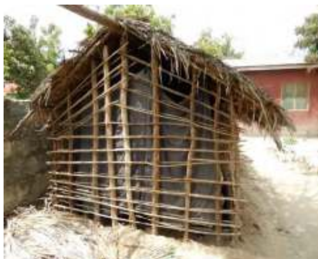
Figure 2: Detail of timber support to a mud house, House 7
