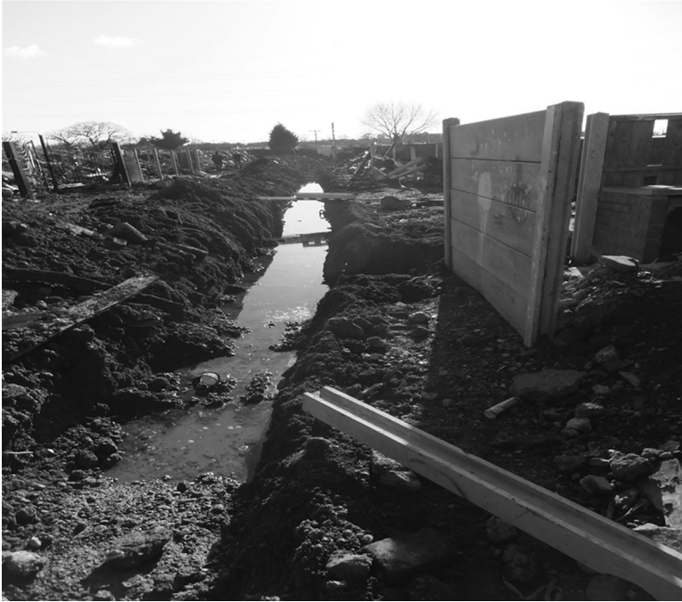
Figure 9.1 Open sewage flows between the Bund Walls at Dale Farm, 2012. Photo by Lynne McCarthy.
