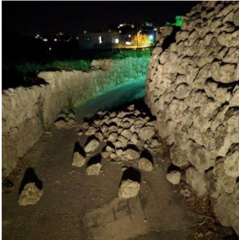
Fig.48 Damaged wall after Ischia Earthquake, August 21, 2017
