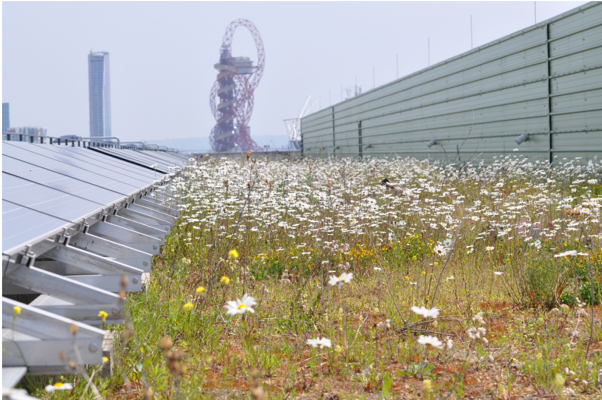
Figure 2. Biodiverse (biosolar) roof in London's Queen Elizabeth Olympic Park. The roof was designed to contribute to targets for Open Mosaic Habitat creation in the Olympic Park Biodiversity Action Plan (BAP). Image © Stuart Connop
