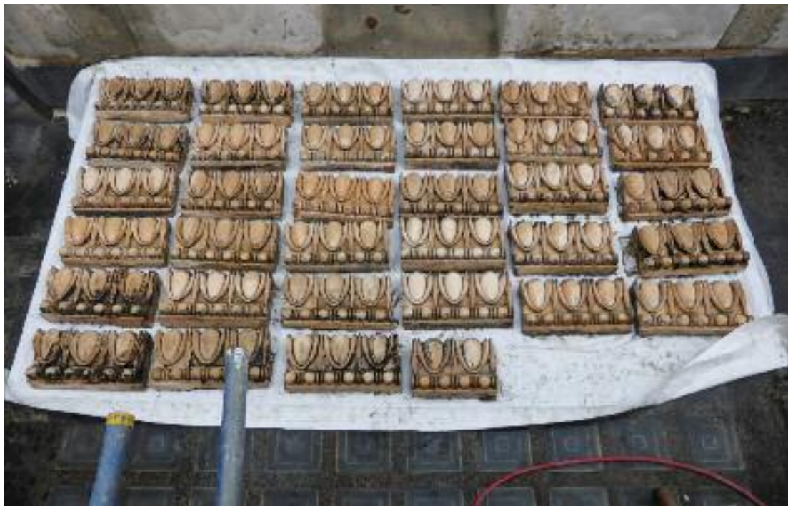
Terracotta elements undergoing cleaning
