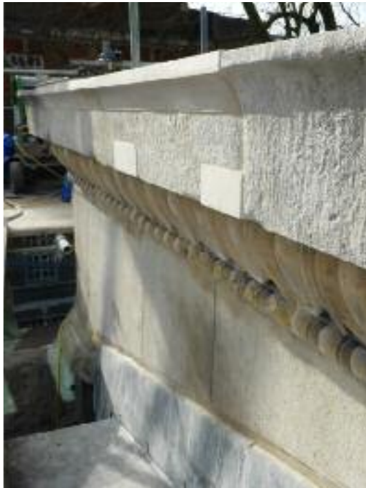
Completed coping edge repair
