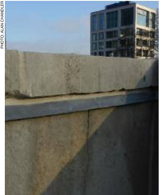
Completed inner parapet walls with cramp repair and lead drip detail
