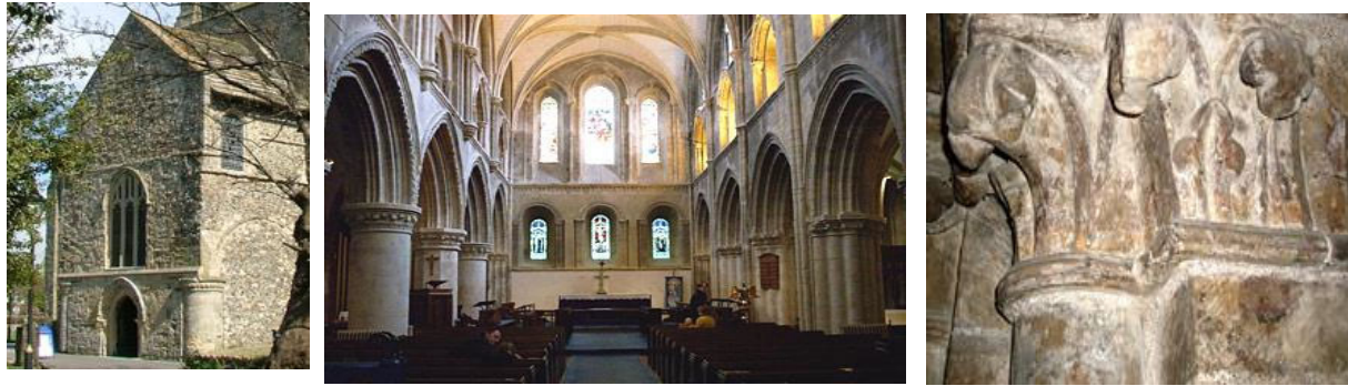
Figure 1: St Mary de Haura Church (left); Internal space of the church (middle); Column with old paint (right)
