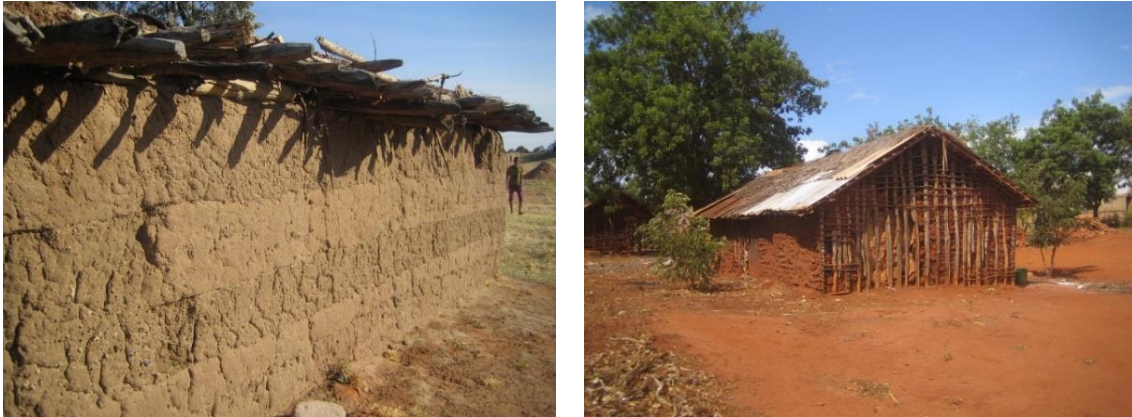
Figure 7. Cob ( left ); Mud and Poles ( right ). Source: The authors.
