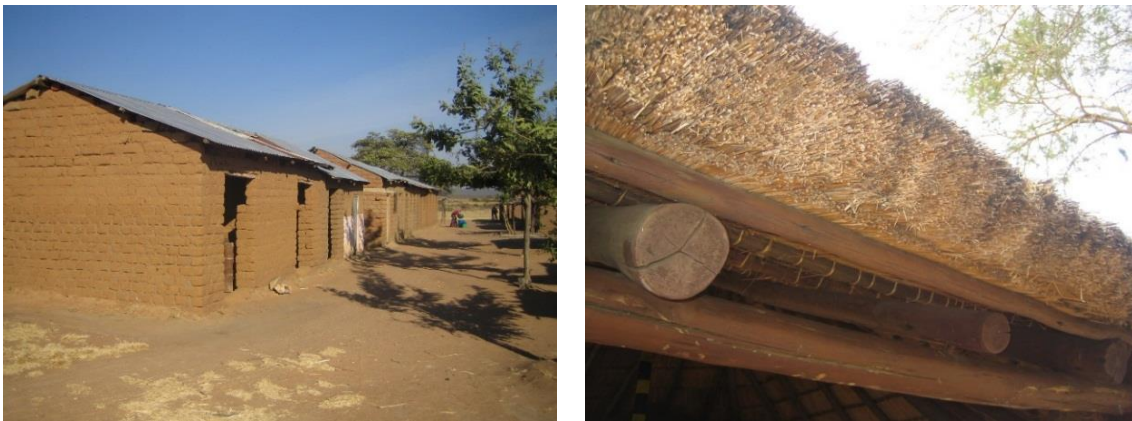
Figure 6. Iron sheet roof ( left ) and thatched roof ( right ). Source: The authors.
