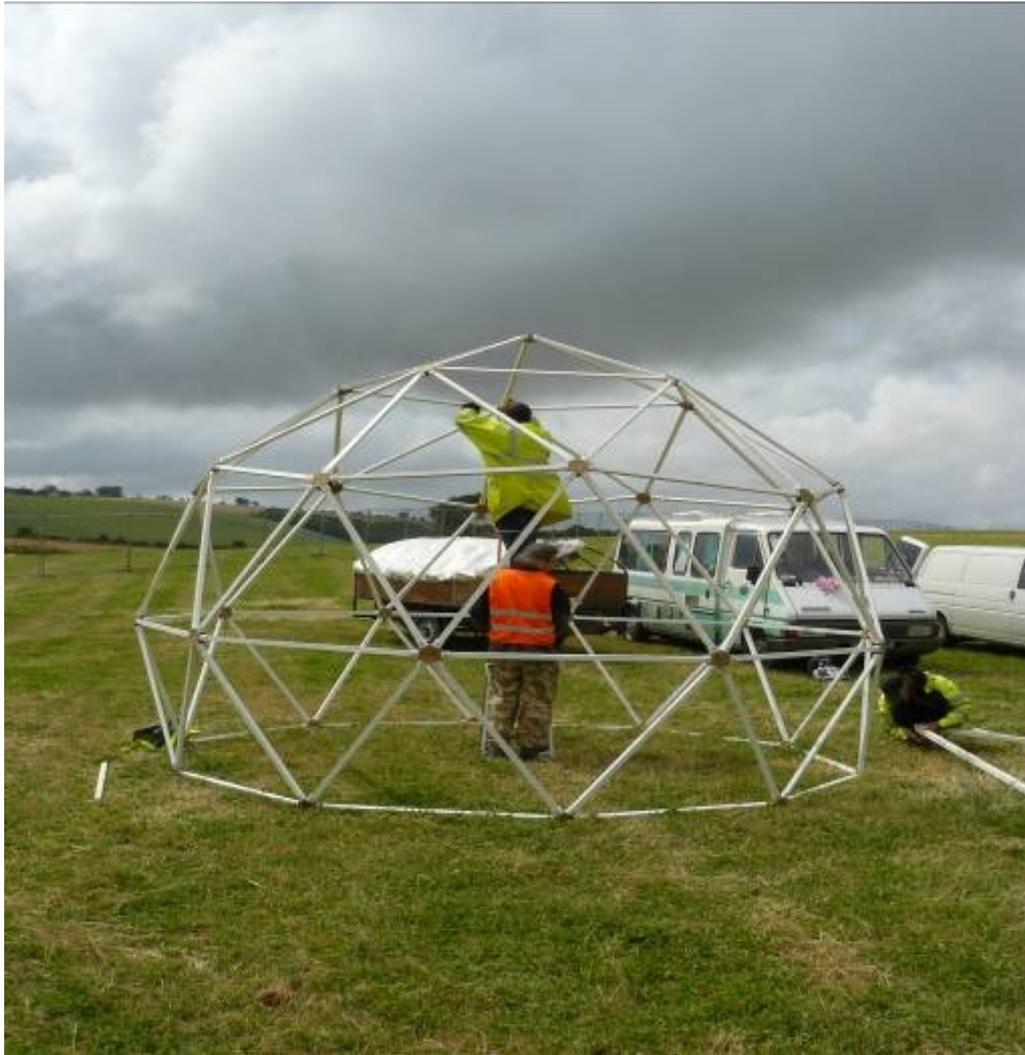
Figure 5: The day before show time, Geo-Lite's Pete Wilson (orange, or darker, jacket) directed Flying Lotus' Alan Turnbull as he connected hubs on the smaller of the psytrance stage two domes. The invisible presence in the dome-erecting team was me, on a steep learning curve. (Photograph Charles de Ledesma, 2008)
