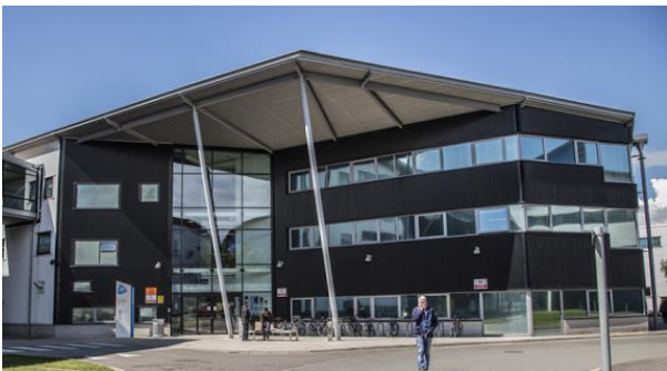
Figure 3: External southeast elevation of the building demonstrating the metal cladding and fenestrations.
