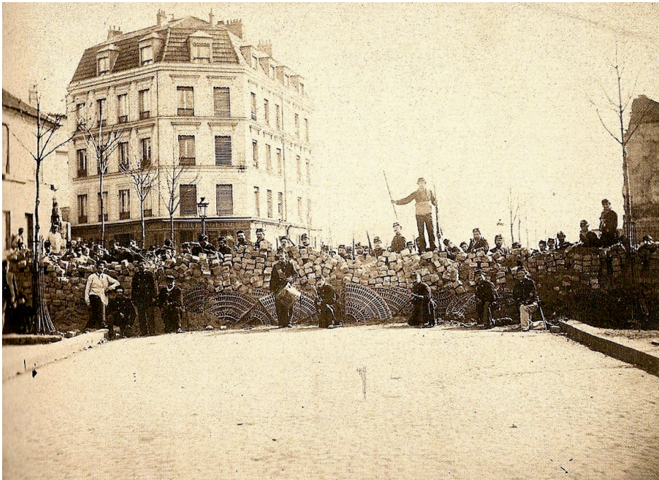
Fig. 2.1. Anonymous: Barricade du Boulevard de Puebla, hauteurs de Ménilmontant 18 mars 1871 . This shows the basic barricade thrown up quite spontaneously and of combined materials including sandbags, paving stones, furniture and interestingly, Haussmann's tree base grills. Despite the hasty erection these barricades—and this one in particular –were often more resistant than the larger barricades.
