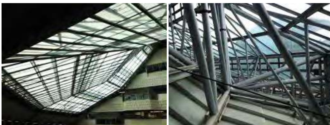
Figure 7: Glazed, double-skin roof of the library
