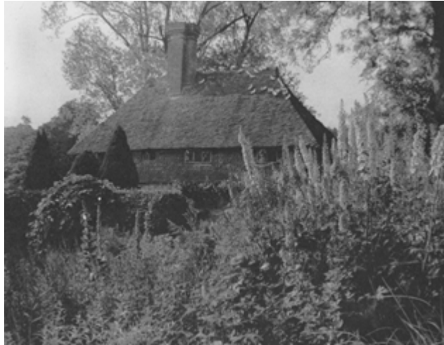
Fig. 8 View towards farm and bathing pool, Valewood Farm, Sussex (1935, CL)
