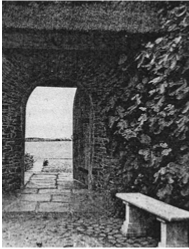
Fig. 33 Entrance, Cock Rock, Croyde, Devon, Oliver Hill, 1925 (Powers, 1989)
