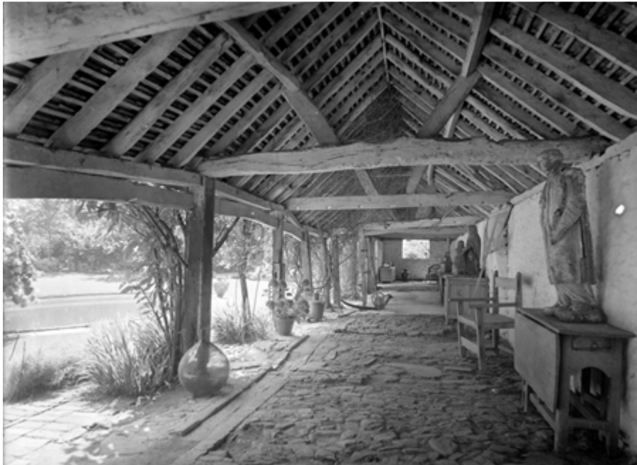
Fig. 27 Converted Byre, Valewood Farm, Sussex, Oliver Hill (1935, CL)
