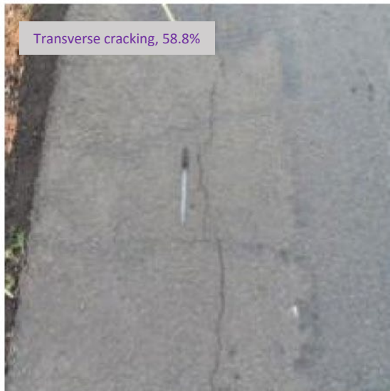
FIGURE 8 Verification of most promising models based on Strategy 3 for transverse cracking
