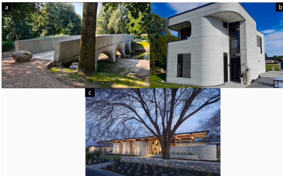
Fig. 12. Examples of projects based on 3DCP: (a) Bridge, Nijmegen, the Netherlands (PERI 3D Construction); (b) Two storey house, Beckum, Germany (PERI 3D Construction); (c) House Zero, East Austin, USA, 2022 (ICON Build).
