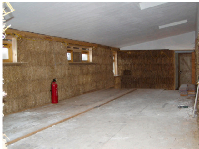
Fig. 7. Load-bearing straw bale wall under construction [59].
