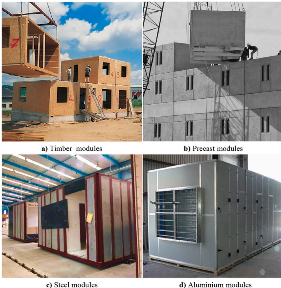
Fig. 11. Prefabricated volumetric modular (PFVM) units with different construction materials [13].
