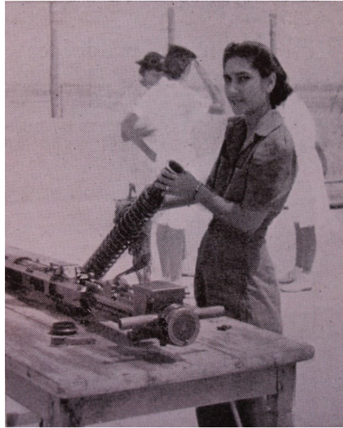
Fig. 30: 'Stripping and Cleaning an Oerlikon Gun', from Wrins and How They Served , 27
