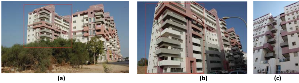
Figure 1. The current condition of the prototype residential tower block development and the south west facing tower block.
