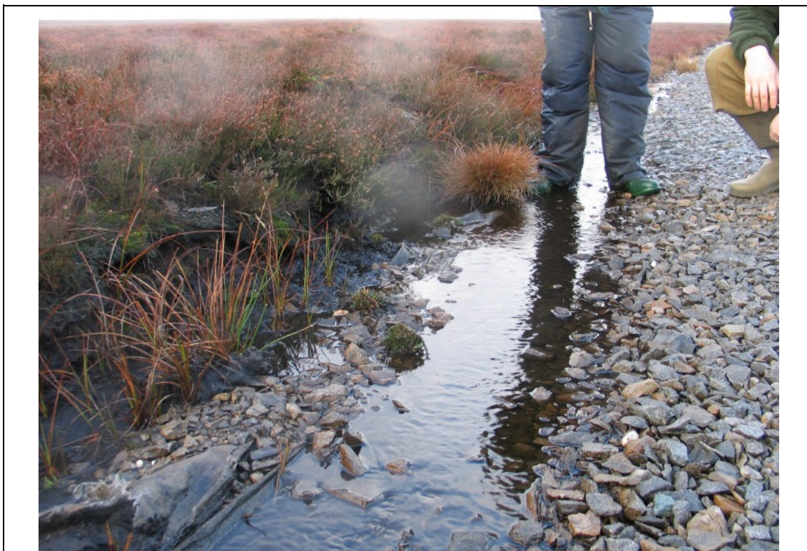
Figure 6. Ponding alongside a floating road.
