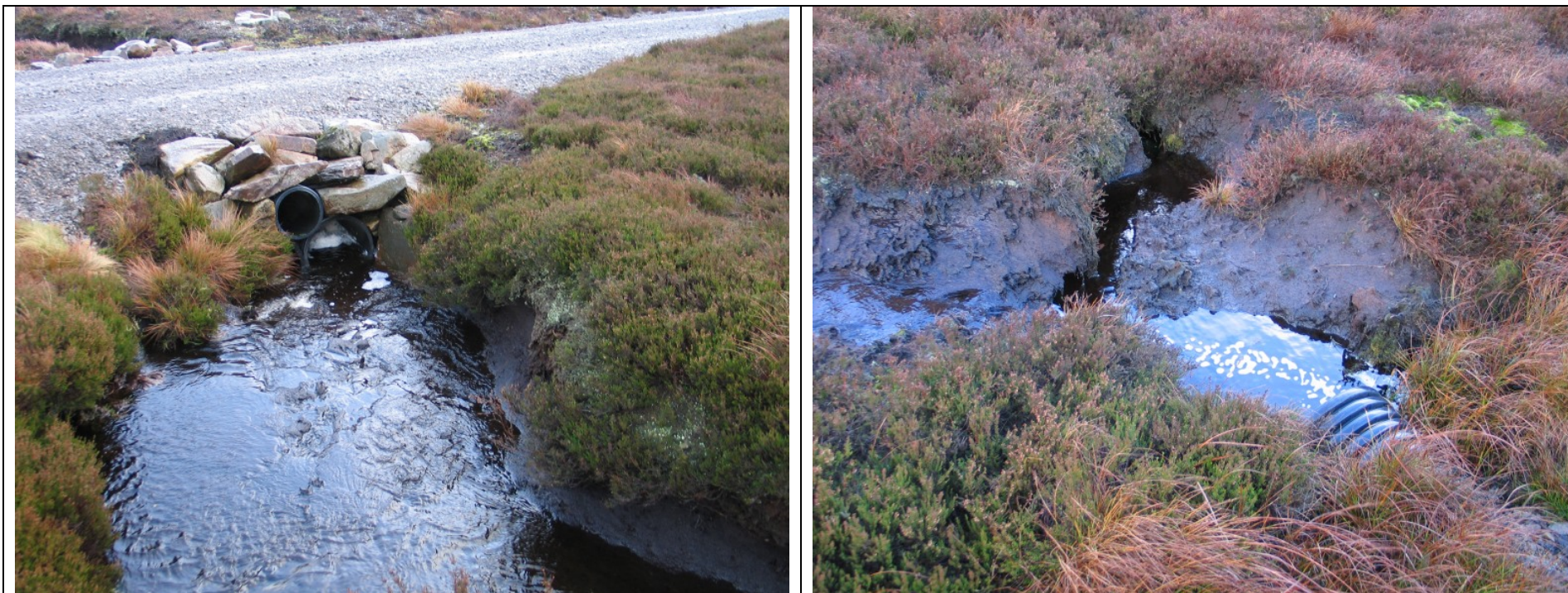
Figure 7. Cross-drains associated with a floating road.
