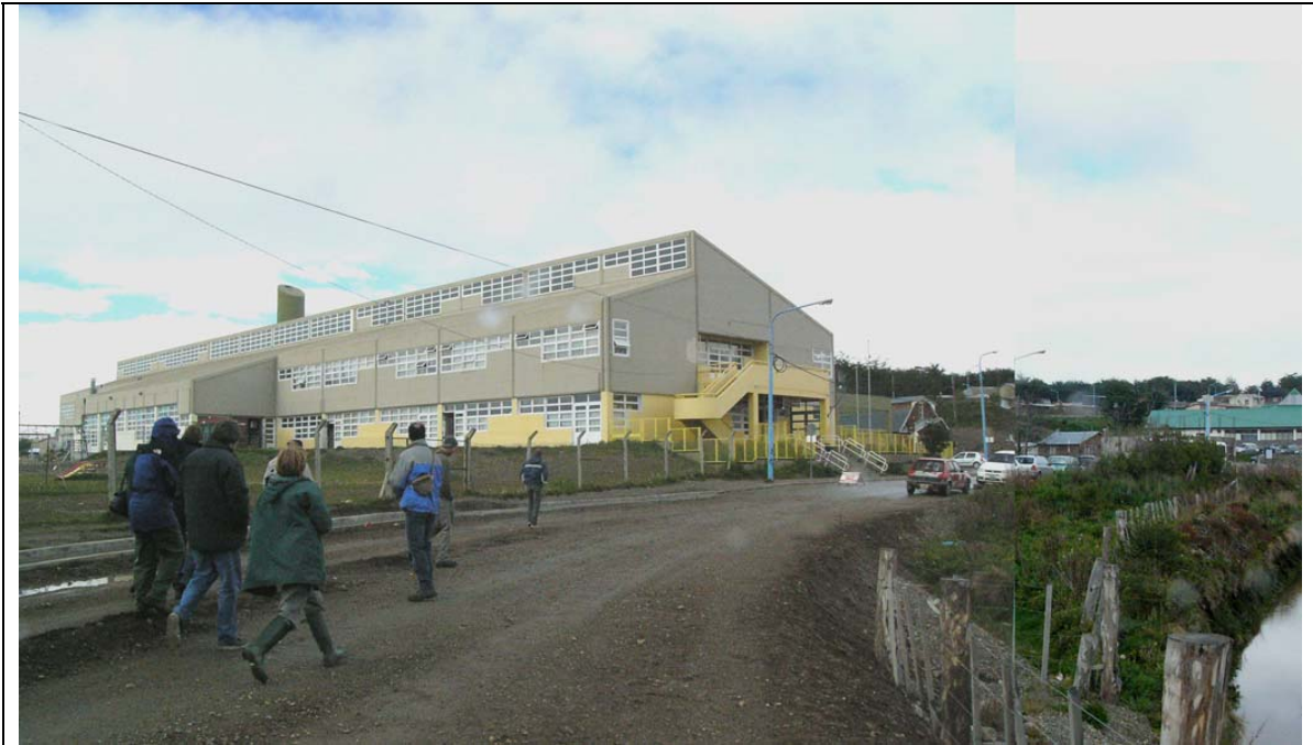
Figure 2. Abandoned school construction project on peat.
