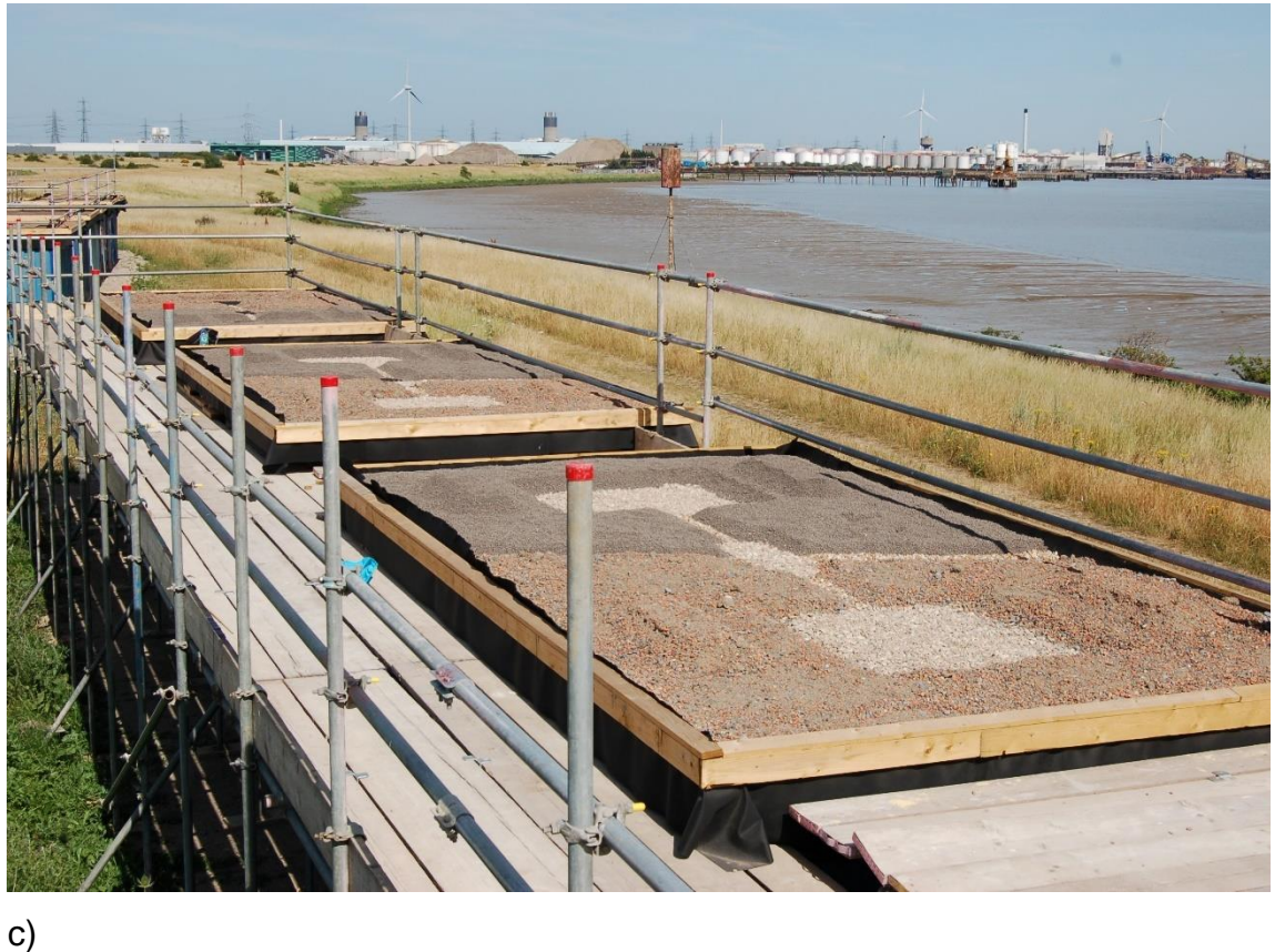
Plate 3.5. Installation of aggregates onto the experimental green roofs, Barking Riverside, East London. (a) wooden frame template used to replicate baseline conditions across all roofs, (b) newly installed aggregates showing mounds and gravel-lined hollows to provide structural diversity and areas for pooling of rainwater, (c) view of roofs once construction was completed prior to planting.
