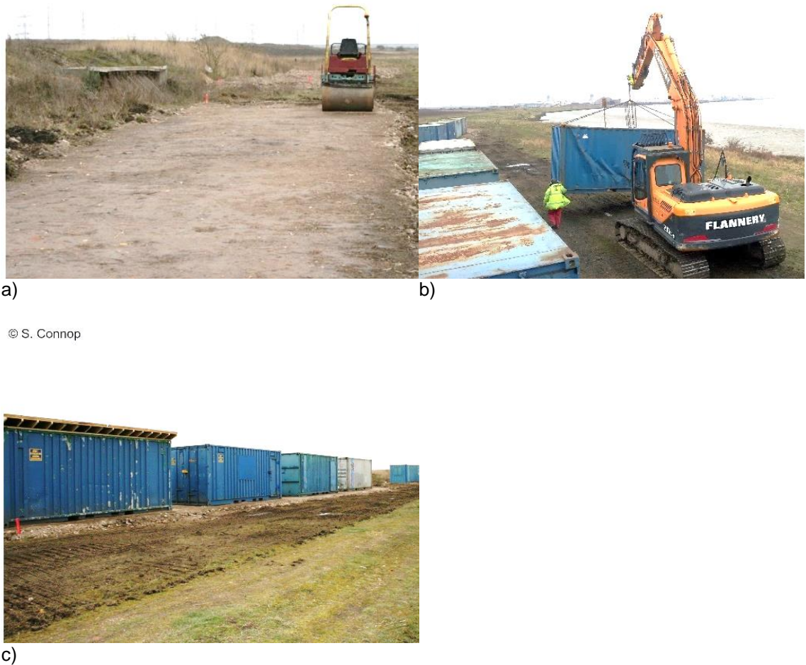
Plate 3.1. Setting up the green roof experiment at Barking Riverside, East London. (a) construction of a levelled hardcore base for containers, (b) excavator moving containers into position, (c) containers in situ with a 2m 'ecological' gap between experimental plots.
