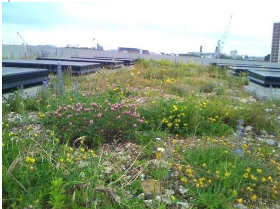
Plate 1.1. Examples of (a) an industry-standard Sedum green roof, and (b) a biodiverse green roof. Image (a) Sedum EGR on Eversheds Sutherland LLP, City of London, EC2; image (b) biodiverse EGR on Laban Dance Centre, Deptford, London SE8. Images © G. Kadas & D. Gedge.
