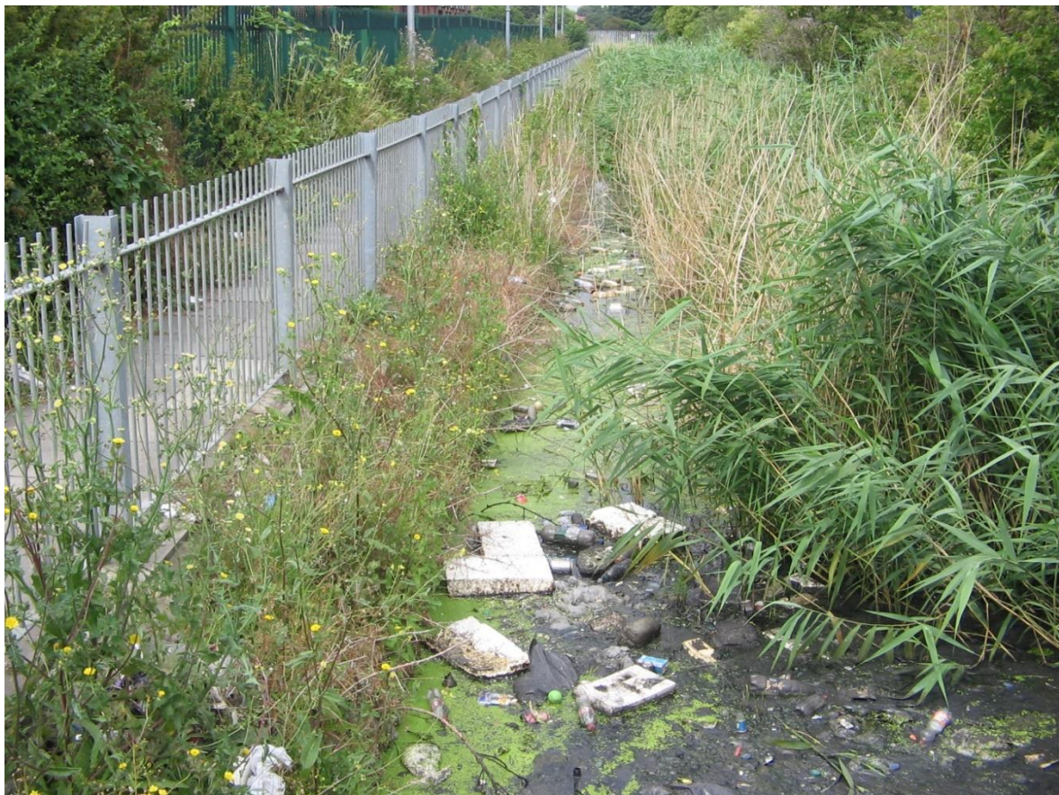
190 Figure 2. Example of a nature-based solution with inadequate stewardship. The stewardship of this stormwater 191 management ditch was not considered in relation to appropriate management. As such, it is seen as a negative 192 feature of the area and is used for dumping of trash. © Stuart Connop
