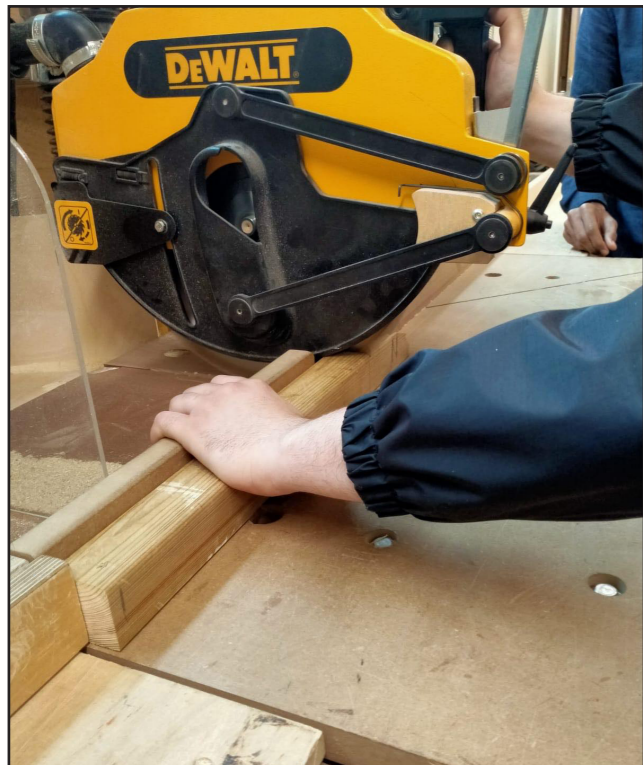
Fig. 62 - CUTTING THE THE BATTENS TO THE RIGHT LENGHT
