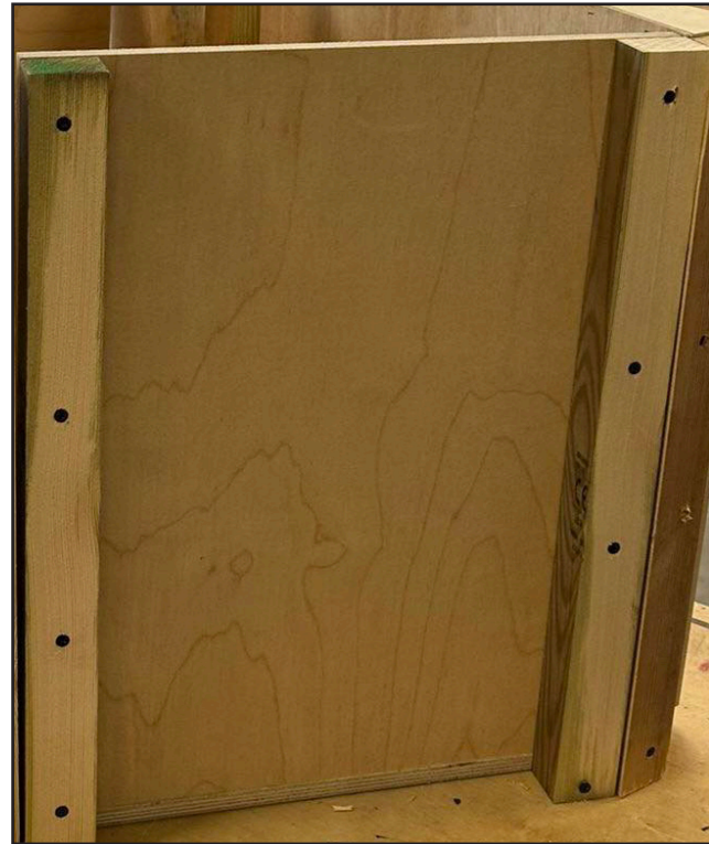
Fig. 61 - SCREWING THE BATTENS INTO THE WALL
