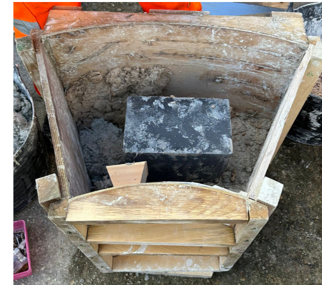
Fig.84 - The void and blocks inside the mould
