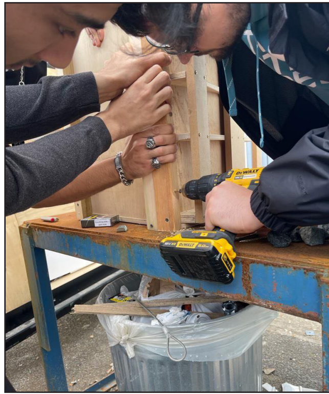
Fig. 74 - SCREWING THE PARTS TOGETHER
