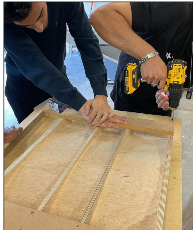
Fig. 56 - SCREWING THE REINFORCEMENT SYSTEM
