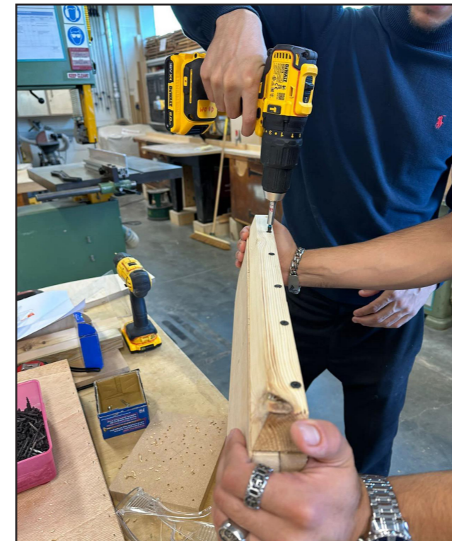
Fig. 65 - SCREWING THE BATTEN INTO THE RIBS
