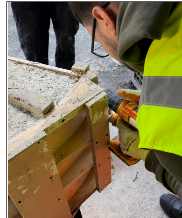
Fig. 91 - UNSCREWING THE CURVES
