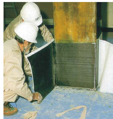
Fig. 1 FRP confinement of concrete columns
