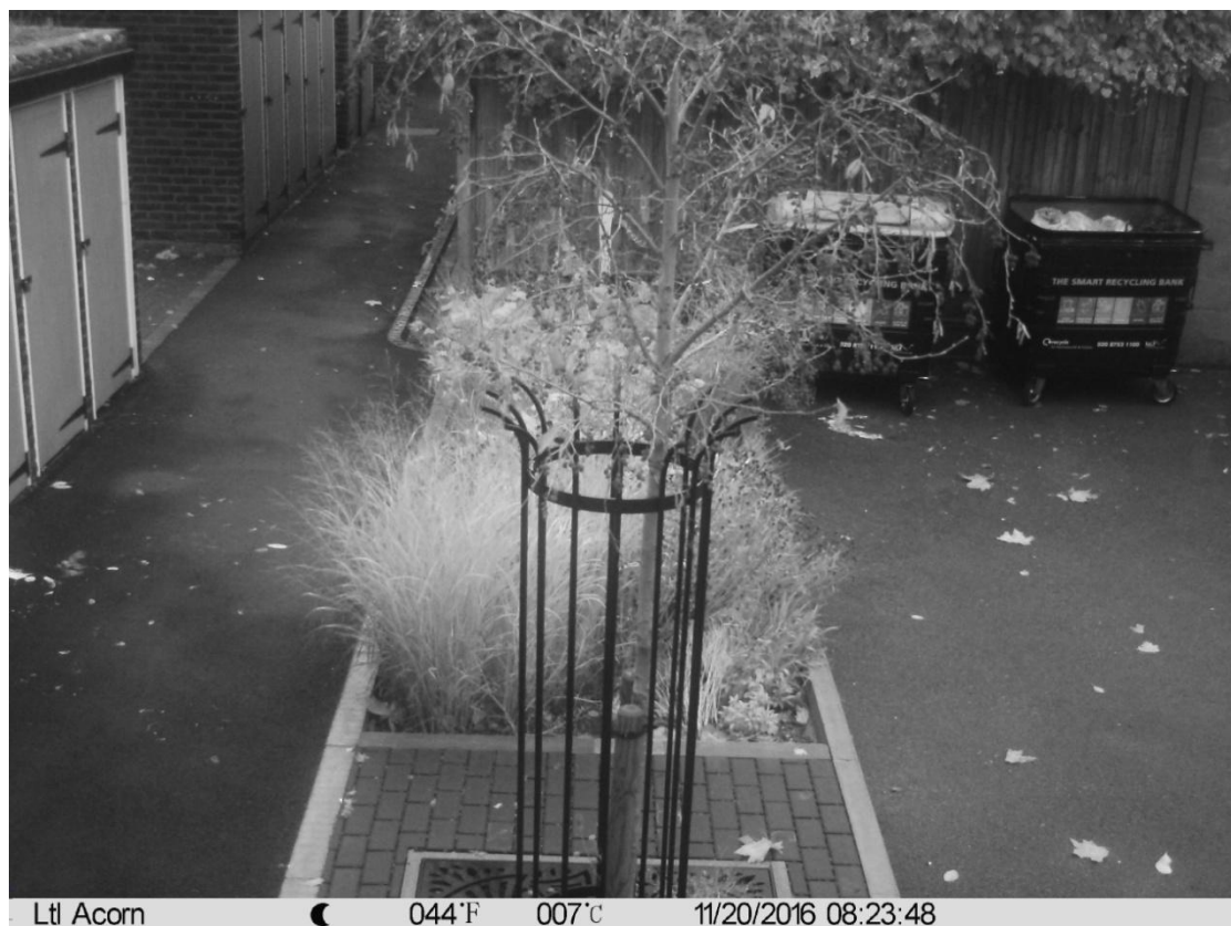
Figure 11. Time-lapse camera images from Richard Knight House rain garden (FPC5), 20/11/2016. Images show i) no evidence of overflowing during period of highest rain intensity at 05:36 and ii) evidence of 100% infiltration/conveyance by the end of the intense rain event at 08:23 on the same day.
