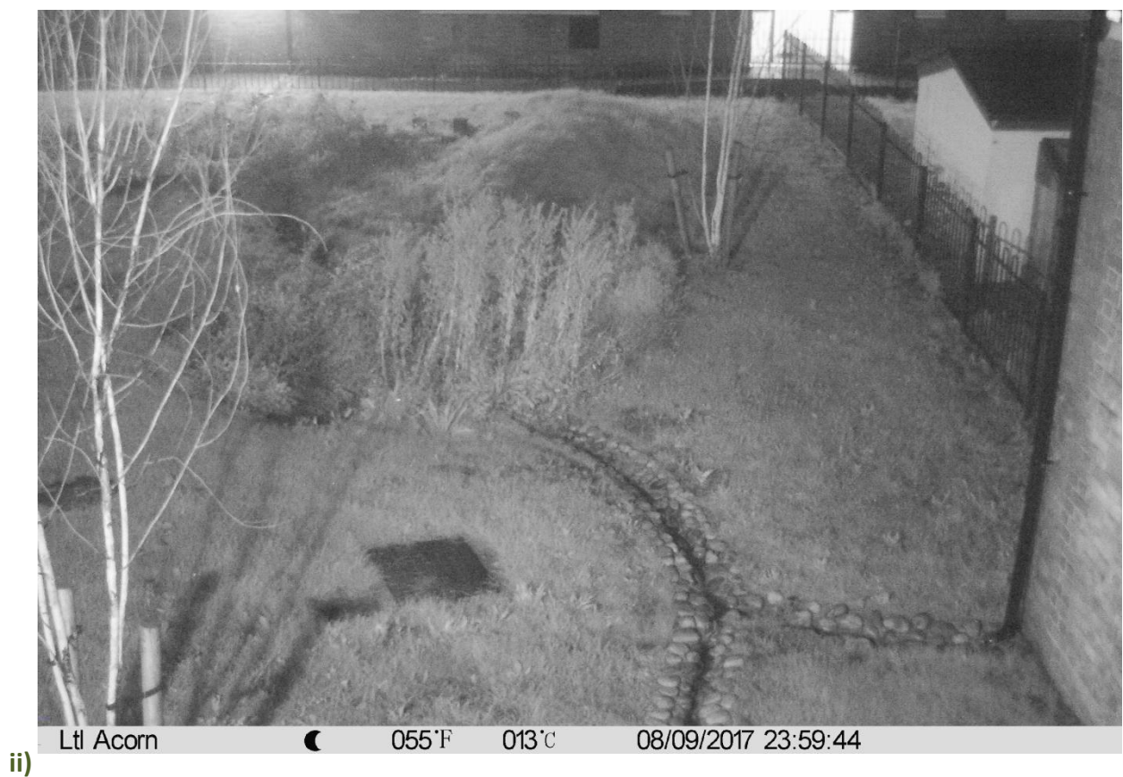
Figure 19. Time-lapse camera images from Community Hall and Sofia House basins (FPC2), 09/08/2017. Images show i) no evidence of overflowing during a period of high rain intensity at 10:48 and ii) evidence of 100% infiltration/conveyance by the end of the intense rain event at 23:59 on the same day.
