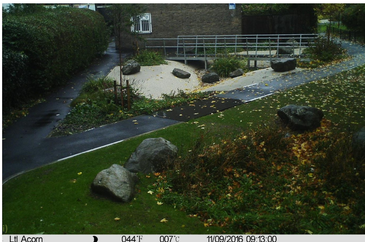
Figure 9. Time-lapse camera images from Adella House grass and stoney basins (FPC3), 09/11/2016. Image shows no evidence of pooling and evidence of 100% infiltration/conveyance towards the end of the prolonged rain event at 09:13.
