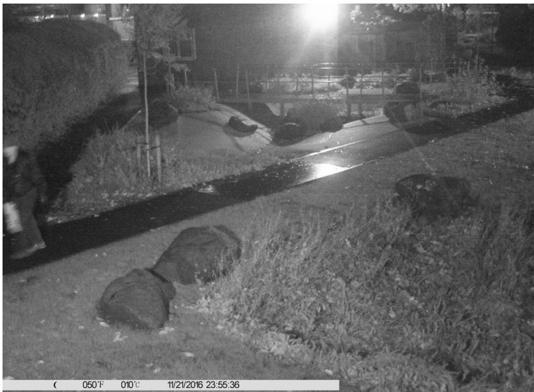
Figure 126. Time-lapse camera images from Adella House grass and stoney basins (FPC3), 21/11/2016. Images show i) no evidence of overflowing during a period of high rain intensity at 14:13 and ii) evidence of 100% infiltration/conveyance by the end of the intense rain event at 23:55 on the same day.
