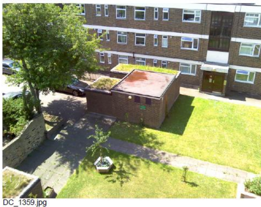
Figure 76. Photo and infrared image of standard pramshed and green roofs at Richard Knight House on the 14th June 2017. FLIR tools software was used to identify temperatures at selected points within the field of view. The hottest temperatures ( >40\text{ }^{\circ}\text{C} ) were associated with the pramshed roof. These areas were recorded as being substantially hotter than the maximum daily temperature recorded by the nearby weather station ( 26.3\text{ }^{\circ}\text{C} ). Temperatures on the pramshed green roofs were substantially lower at <30\text{ }^{\circ}\text{C} . These temperatures were either lower or similar to the temperature of pooled water on the standard pramshed roof ( 29.8\text{ }^{\circ}\text{C} ).
