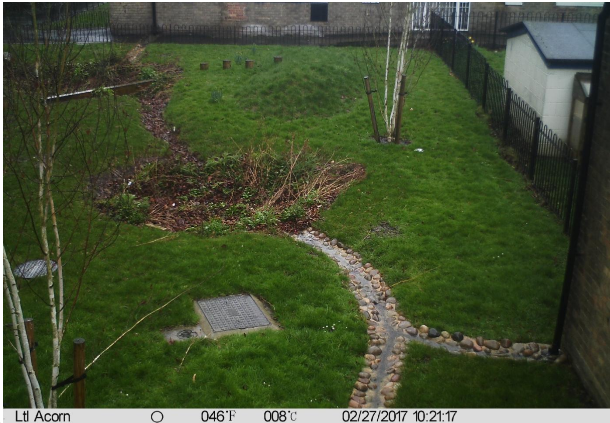
Figure 130. Time-lapse camera images from Community Hall and Sofia House basins (FPC2), 27/02/2017. Images show i) no evidence of overflowing during the first a period of heavy rain at 03:44 and ii) evidence of 100% infiltration/conveyance during the second intense rain event at 10:20 on the same day.
