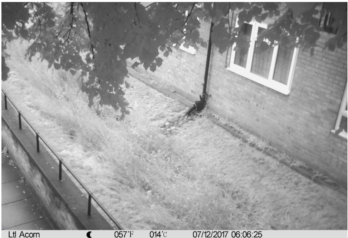
Figure 156. Time-lapse camera images from Beatrice House swale (FPC4), 11/07/2017 and 12/07/2017. Images show i) no evidence of overflowing during a period of high rain intensity at 20:06 on the 11th and ii) evidence of 100% infiltration/conveyance by the end of the intense rain event at 06:06 on the 12th.
