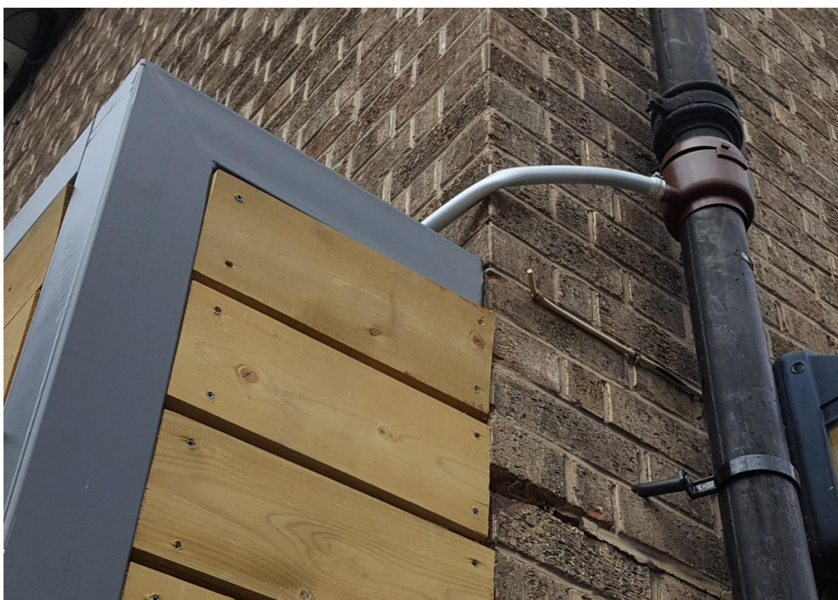
Figure 88. Stormwater interception mechanism that takes rainwater from the downpipe of Mary House and fills the vertical rain garden storage tank, Queen Caroline Estate, 2017. The vertical rain garden comprised a green wall, stormwater storage tank and green facade.
