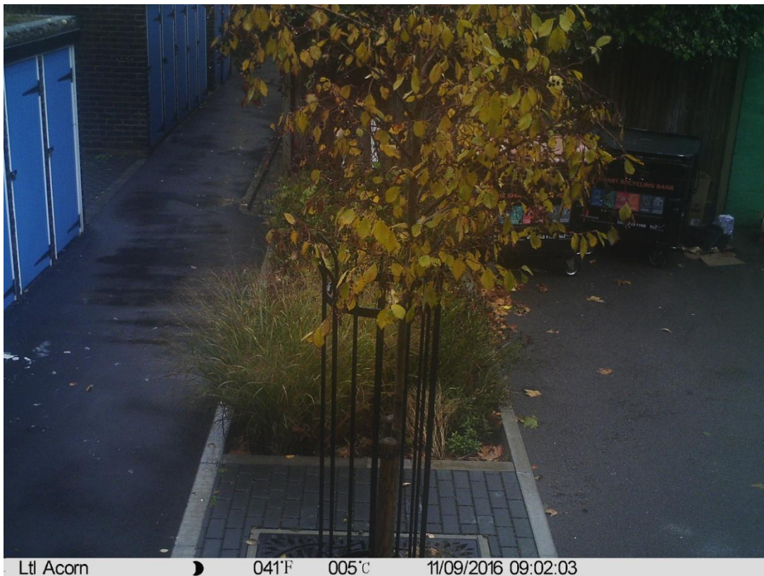
Figure 6. Time-lapse camera images from Richard Knight House swale (FPC5), 09/11/2016. Images show i) no evidence of overflowing during period of highest rain intensity at 06:40 and ii) evidence of 100% infiltration/conveyance by the end of the intense rain event at 09:02 on the same day.
