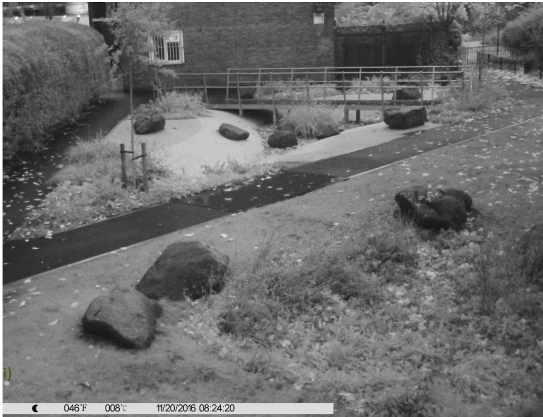
Figure 14. Time-lapse camera images from Adella House grass and stoney basins (FPC3), 20/11/2016. Image shows no evidence of pooling and evidence of 100% infiltration/conveyance towards the end of the prolonged rain event at 08:24.
