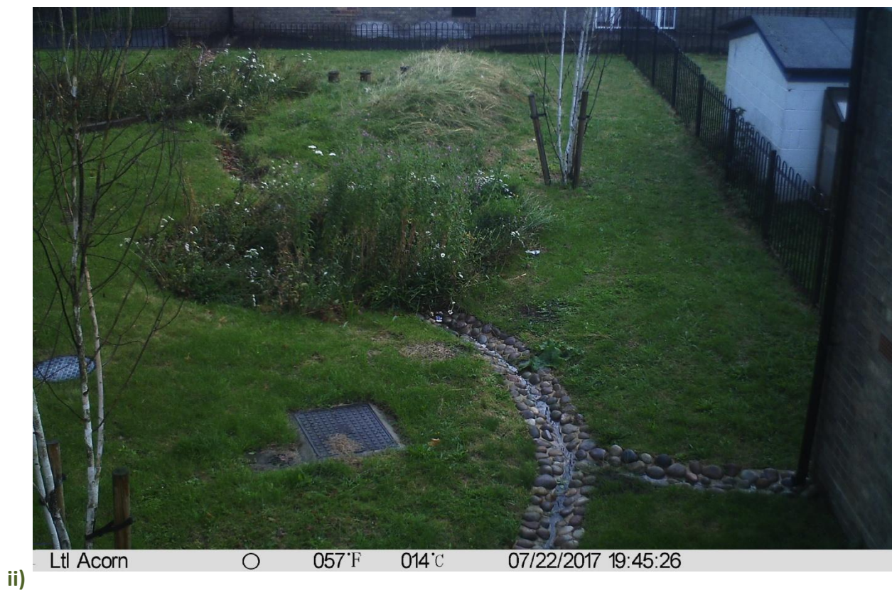
Figure 146. Time-lapse camera images from Community Hall and Sofia House basins (FPC2), 22/07/2017. Images show i) no evidence of overflowing during a period of high rain intensity at 02:18 and ii) evidence of 100% infiltration/conveyance by the end of the intense rain event at 19:45 on the same day.
