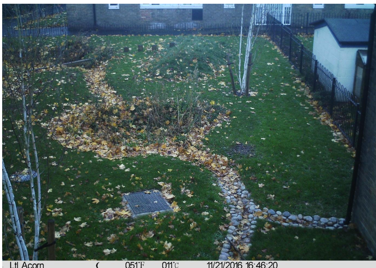
Figure 125. Time-lapse camera images from Community Hall and Sofia House basins (FPC2), 21/11/2016. Images show i) no evidence of overflowing during a period of high rain intensity at 13:52 and ii) evidence of 100% infiltration/conveyance by the end of the intense rain event at 16:46 on the same day.
