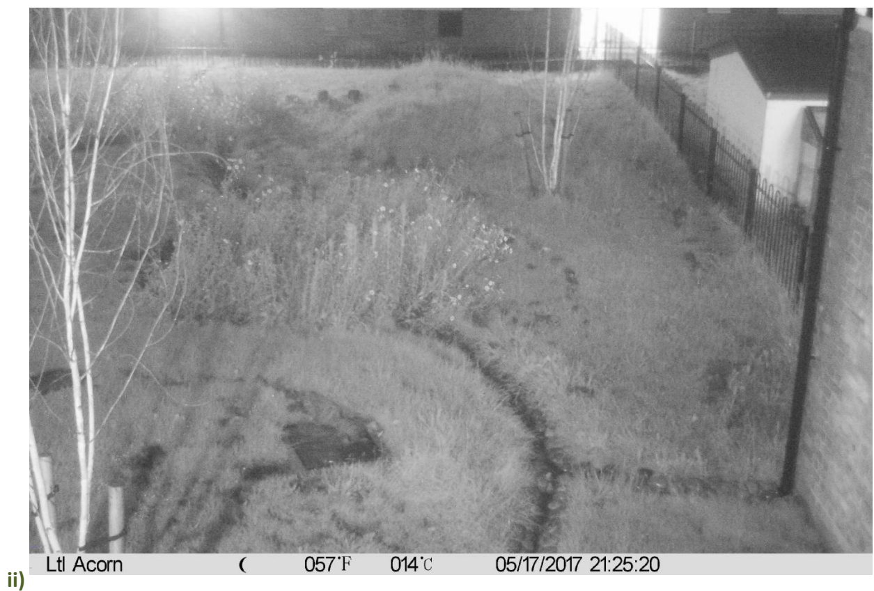
Figure 27. Time-lapse camera images from Community Hall and Sofia House basins (FPC2), 17/05/2017. Images show i) no evidence of overflowing during a period of high rain intensity at 03:32 and ii) evidence of 100% infiltration/conveyance by the end of the intense rain event at 21:25 on the same day.
