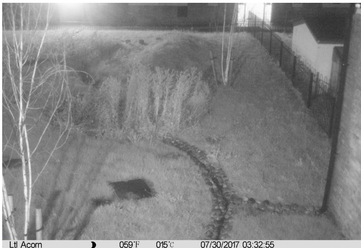
Figure 138. Time-lapse camera images from Community Hall and Sofia House basins (FPC2), 30/07/2017. Images show i) no evidence of overflowing during a period of high rain intensity at 02:18 and ii) evidence of 100% infiltration/conveyance by the end of the intense rain event at 03:32 on the same day.
