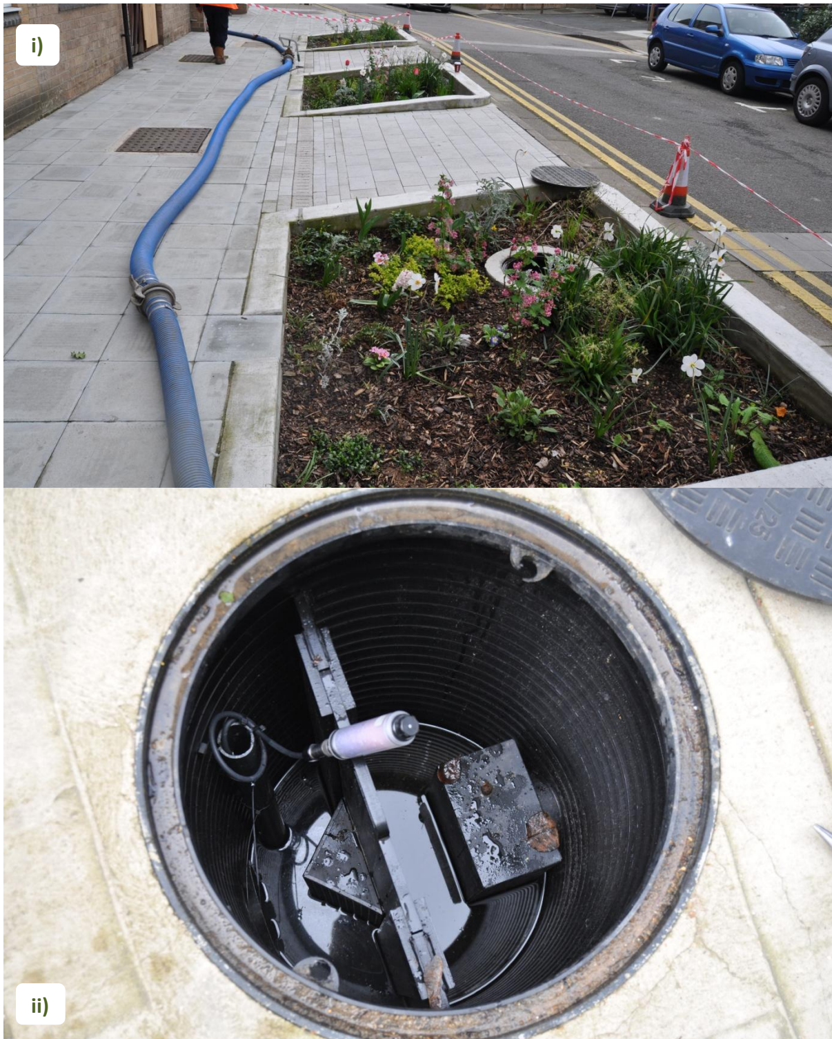
Figure 70. Images from the storm simulation event at the Sun Road rain gardens, Cheeseman Terrace Estate, 24th March 2017. Images show i) Cheeseman Terrace Estate rain gardens before rain simulation; ii) pressure sensor installed in the control flow chamber in the outlet from the rain garden.
