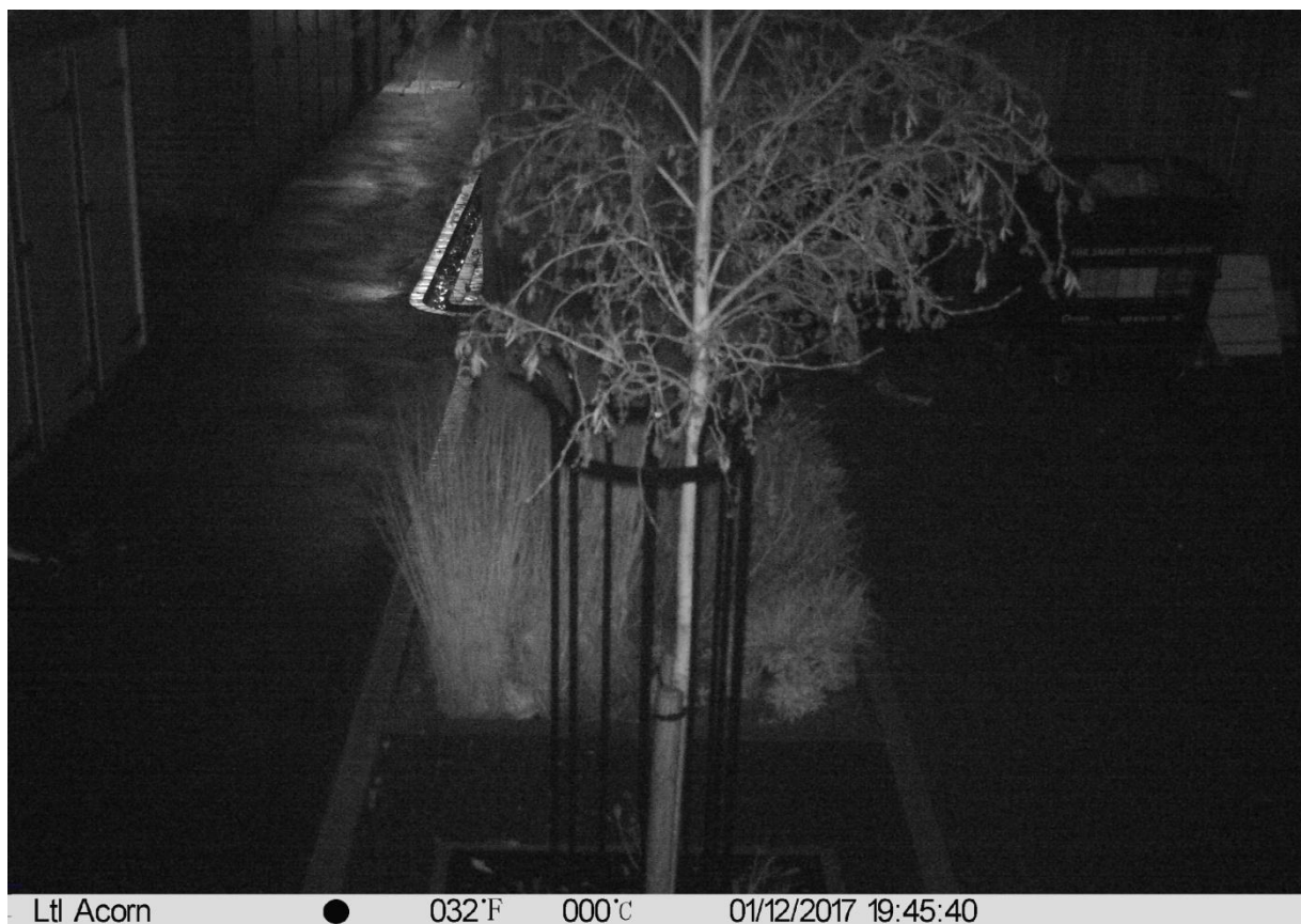
Figure 115. Time-lapse camera images from Richard Knight House rain garden (FPC5), 12/01/2017. Images show i) no evidence of overflowing during period of highest rain intensity at 16:20 and ii) evidence of 100% infiltration/conveyance by the end of the intense rain event at 19:45 on the same day.
