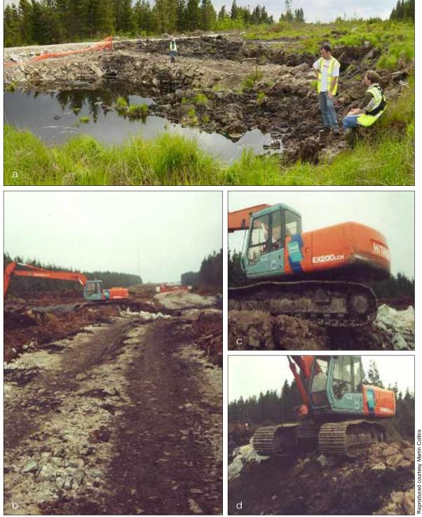
Plate 8.2: The head of the peat slide at T68. a: turbine base excavation in June 2004; b: deformation of floating road October 2003; c, d: an excavator after the bog slide.
