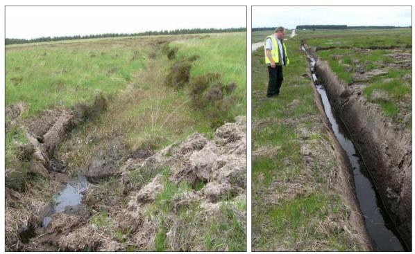
Plate 3.6: Turbary fields on the summit if the site showing (above) an old peat bank and (right) the downslope catchwater drainage system, re-excavated after peat slide in 2003).
