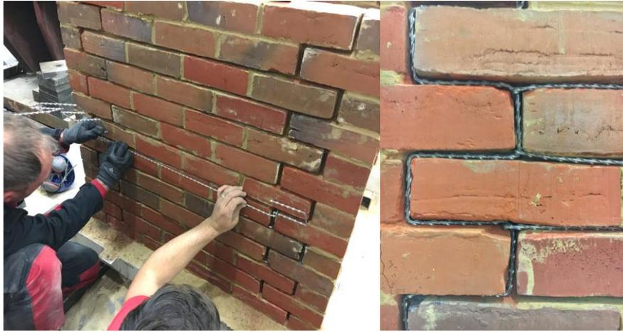
**Fig. 9.** Retrofitted helical bars, wiggled to both bed joints and head joints.
