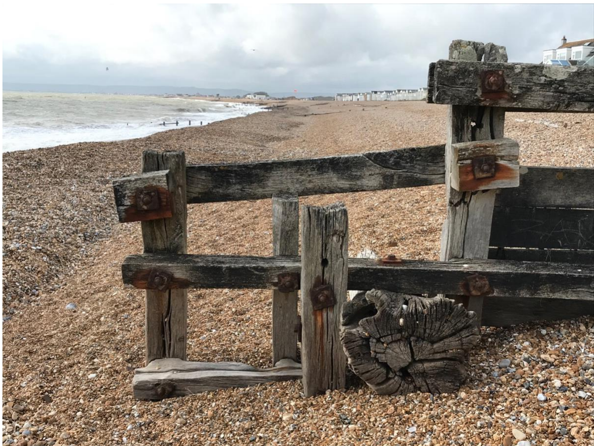
Figure 54: Groyne , 2020, Cooden Beach. Photograph: K J J Warren
