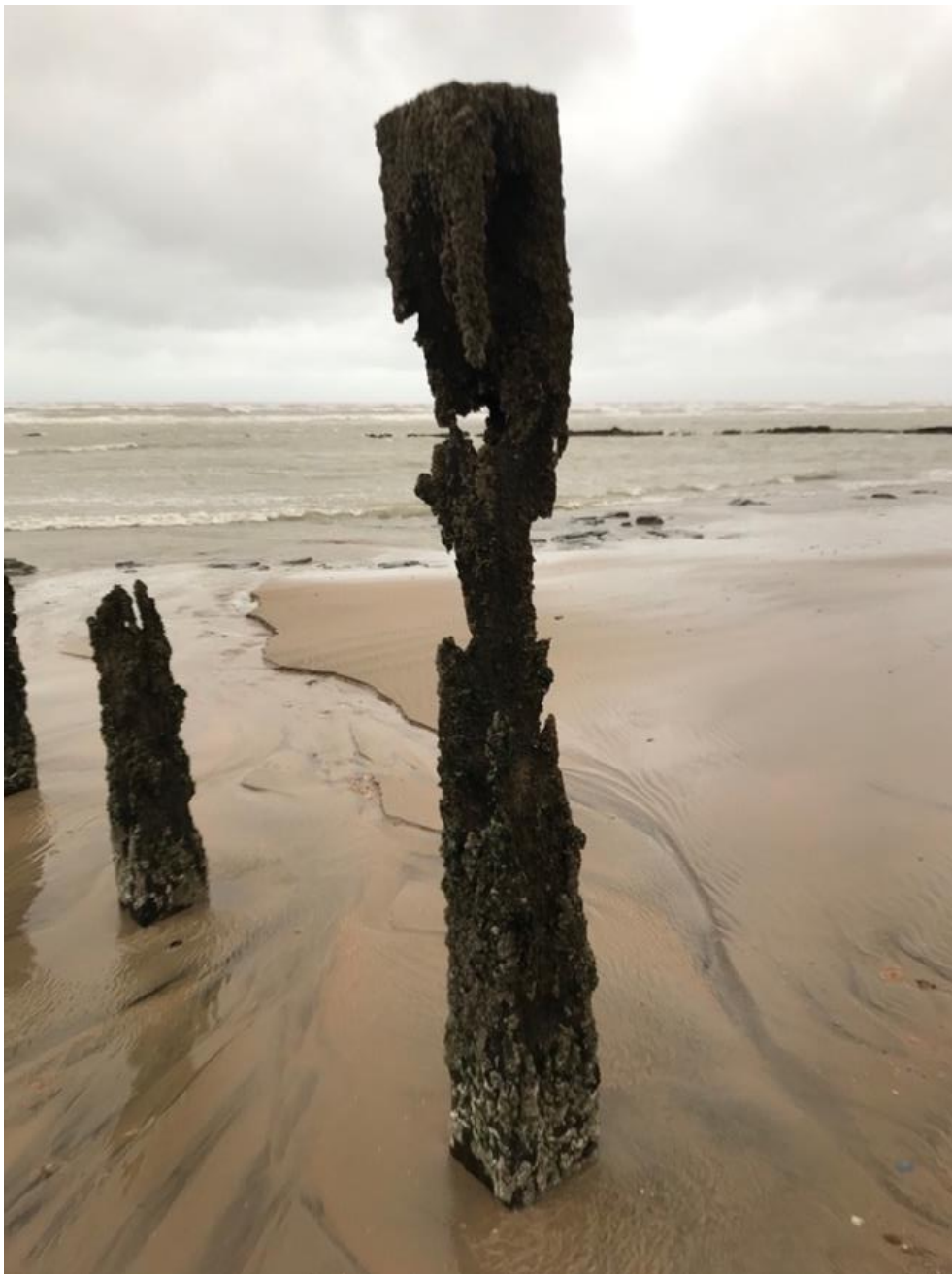
Figure 21: (non) groyne , Cooden Beach, 2020. Photograph: K J J Warren
