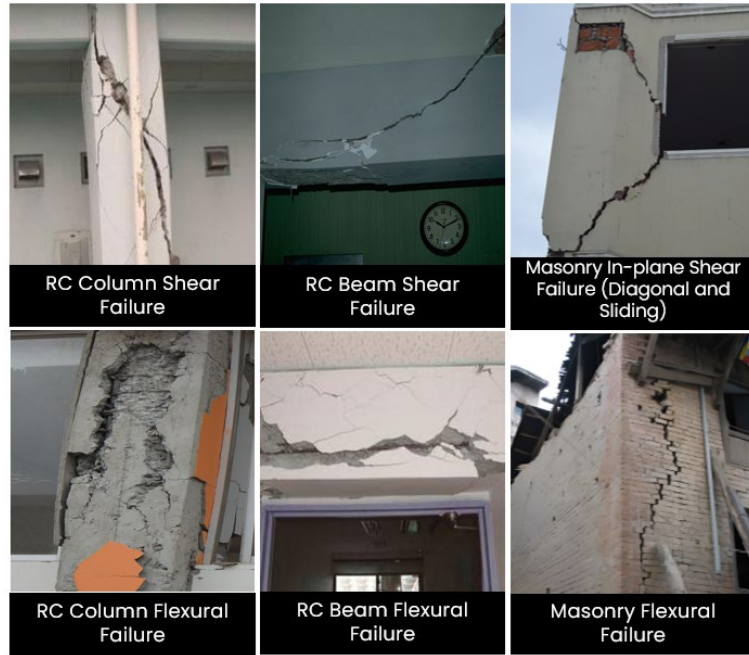
Figure 3: Sample images of shear failure and flexural failure of RC column, RC beam and masonry infill walls included in the database developed in this paper
