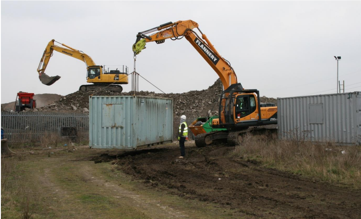
Figure 8. Freight container being moved into position by excavator for the Phase 2 green roof experiment at Barking Riverside, East London.
