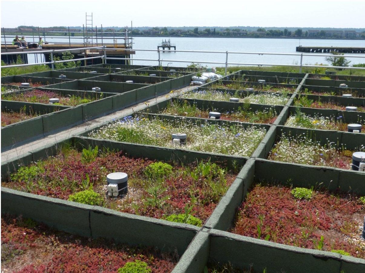
Figure2. Installed green roof test bays at Barking Riverside Offices.
